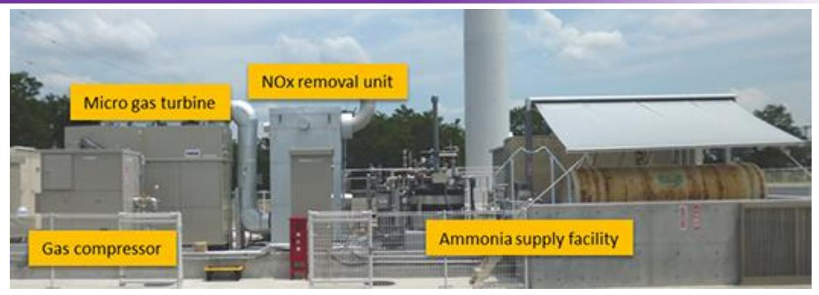
41.8 kW power generation by ammonia/air gas turbine (Japan, 2015) Kurata, et al., PCI 36 (2017) 3351-3359 Kobayashi, et al., PCI 37 (2019) 109-133
