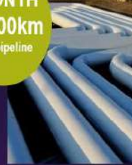
1.4m dia pipe @100bar
