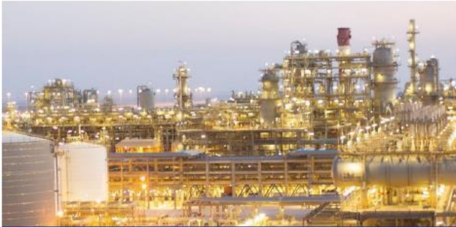
PEARL GTL, QATAR
