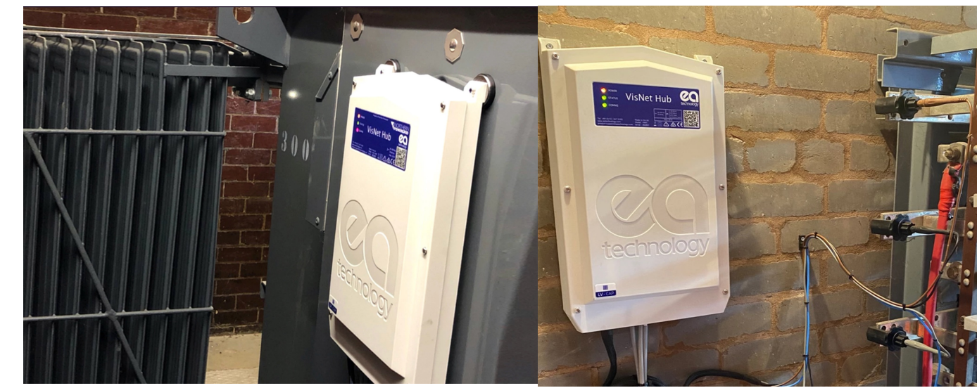
Figure 1: Images of VisNet® Hub installed in a substation
